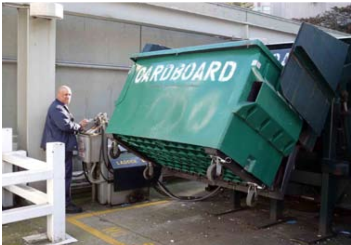
Large compactors are located at each of the Center’s two loading docks.
