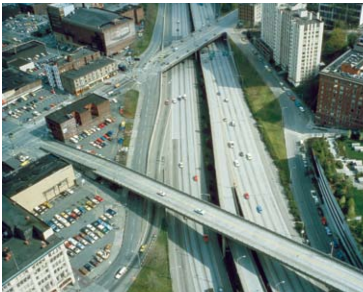
The Convention Center site prior to construction...
