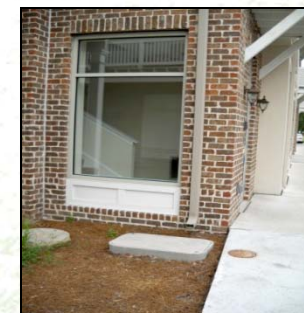
Some of the impervious cover relief comes through design features. The patio at Captain Woody’s is highly pervious, while this downspout sends water into planter areas, not the street system.
