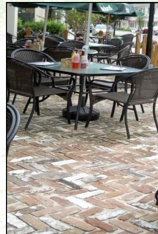
Some of the impervious cover relief comes through design features. The patio at Captain Woody’s is highly pervious, while this downspout sends water into planter areas, not the street system.
