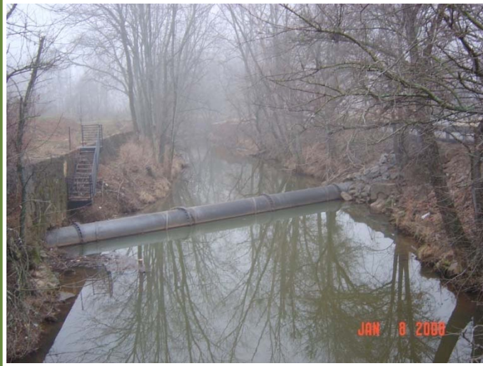
Sewer pipes crossing rivers
