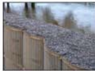
Cedar Rapids' interim flood protection system reinforces the City's current levees with sand and sand-filled temporary barriers.
