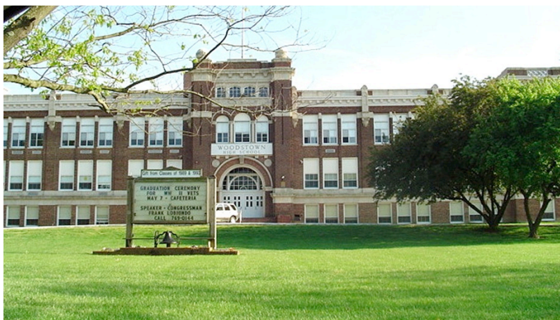
School Biomass Boilers
