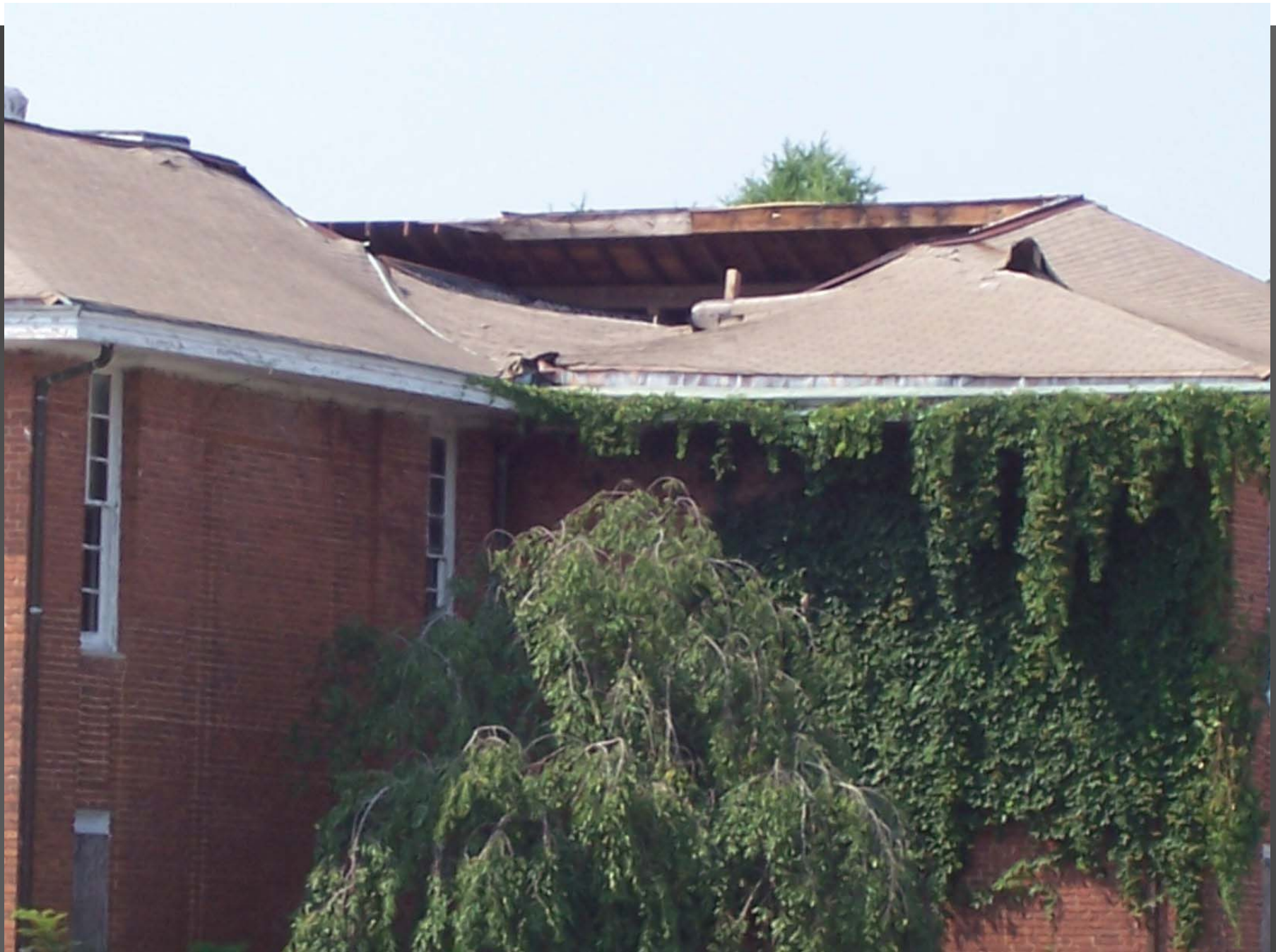
Mayworth School, Cramerton - Before
