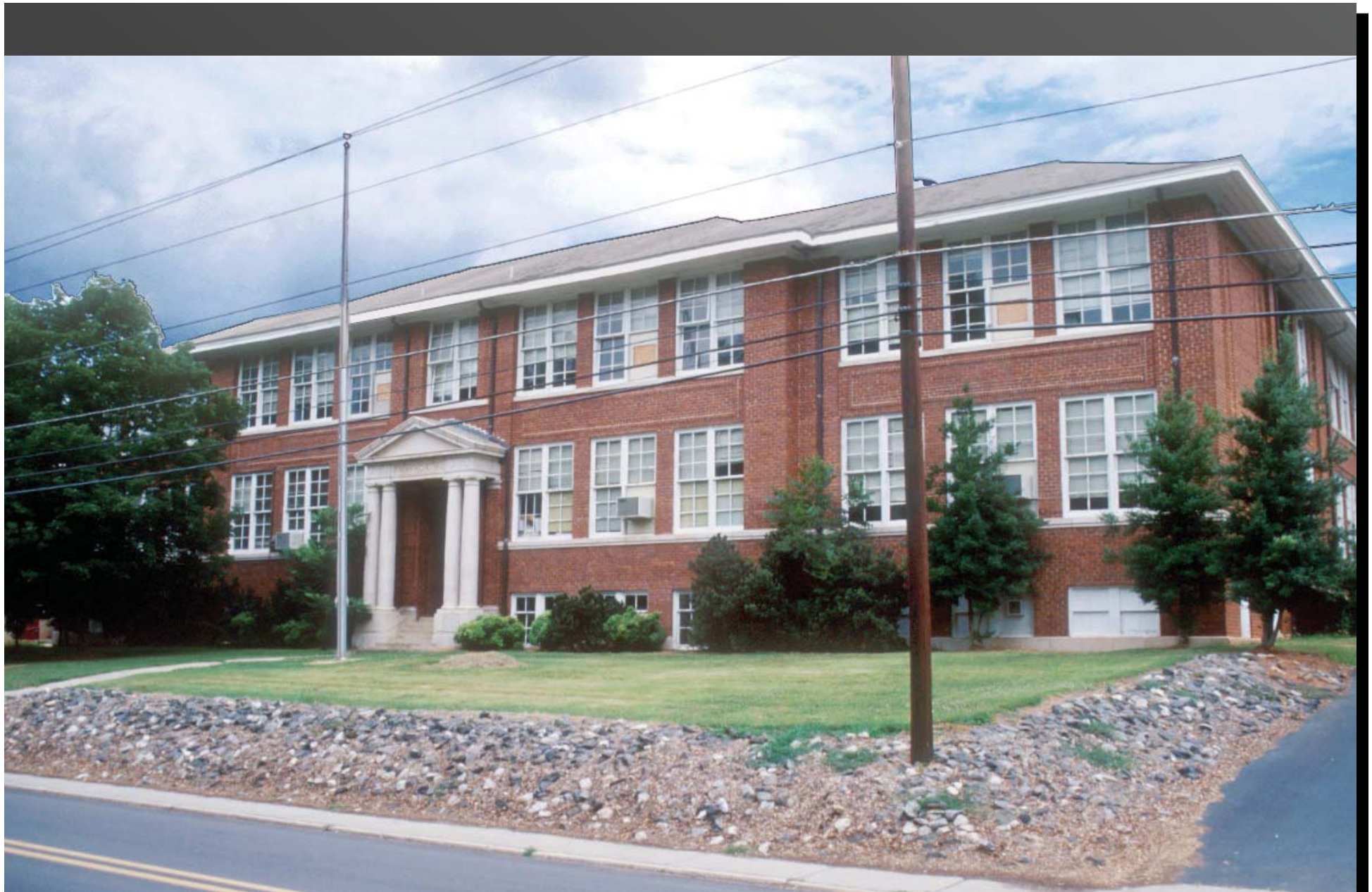
Mayworth School, Cramerton - Before
