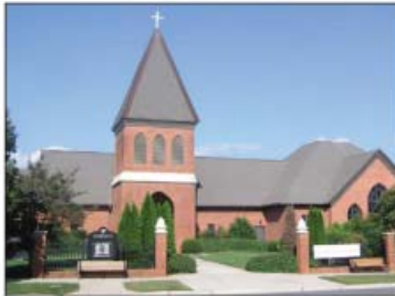
St. Albans Church is a civic building type in New Neighborhood in Old Davidson.
