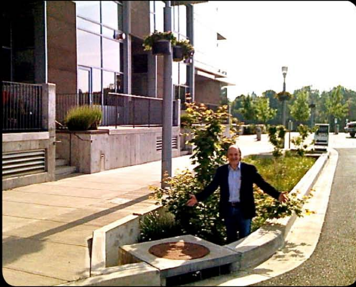
LOW IMPACT URBAN ENVIRONMENT URBAN MOAT TO MANAGE STORMWATER RUNOFF
