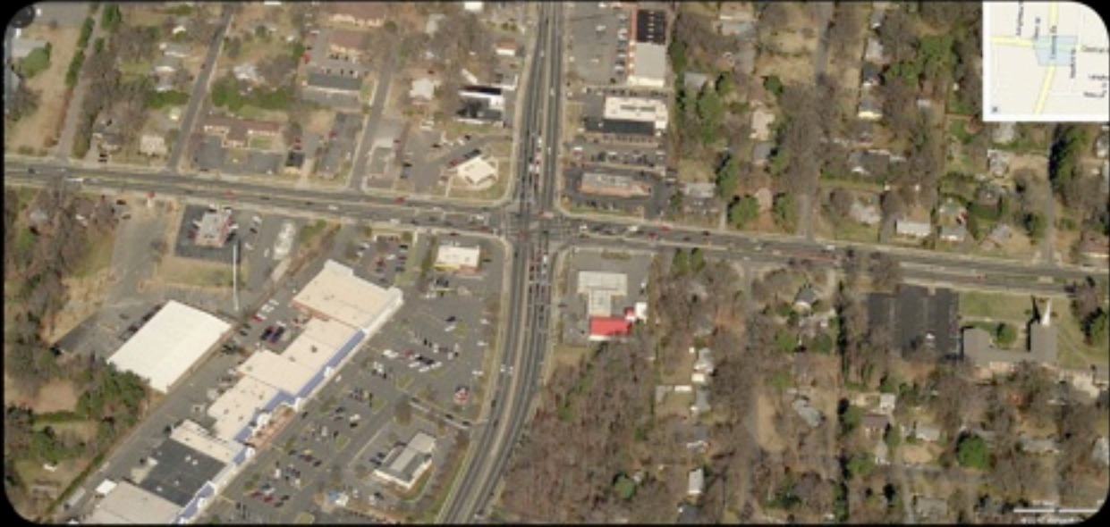
EXISTING SPRAWL INTERCHANGE ALONG THE STREETCAR ROUTE
