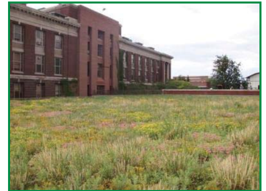
Green Roof at SUNY ESF
