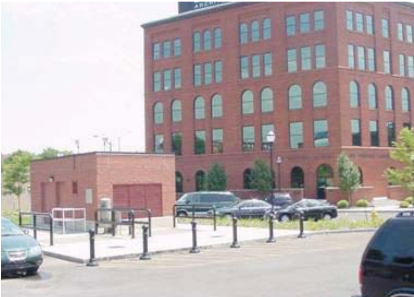
Floatables Control Access Building in Parking Lot
