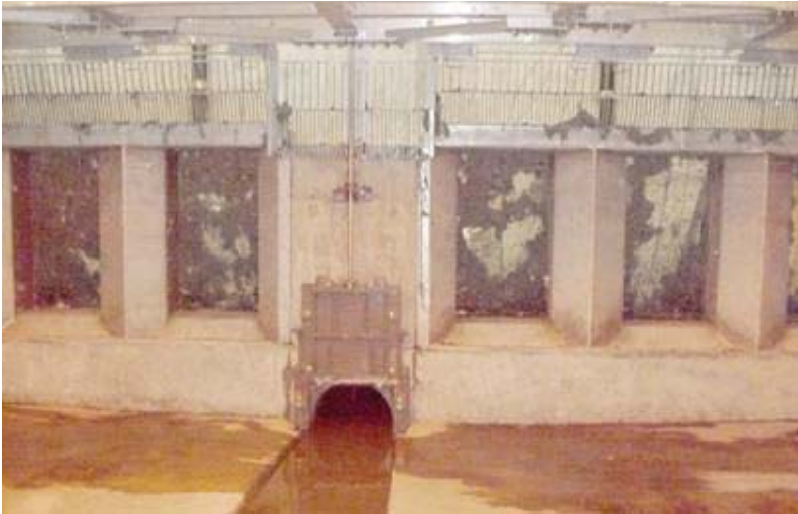
Underground floatables collection chamber
