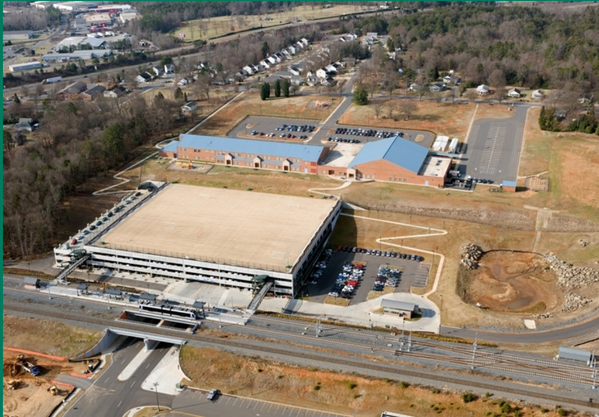
Sterling school/transit parking structure
