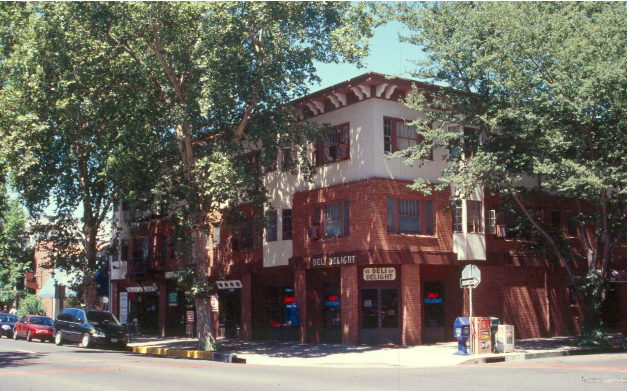
Housing over retail shops
