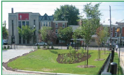
A bioretention area in Wilmington, Delaware, designed to absorb and retain stormwater runoff.
