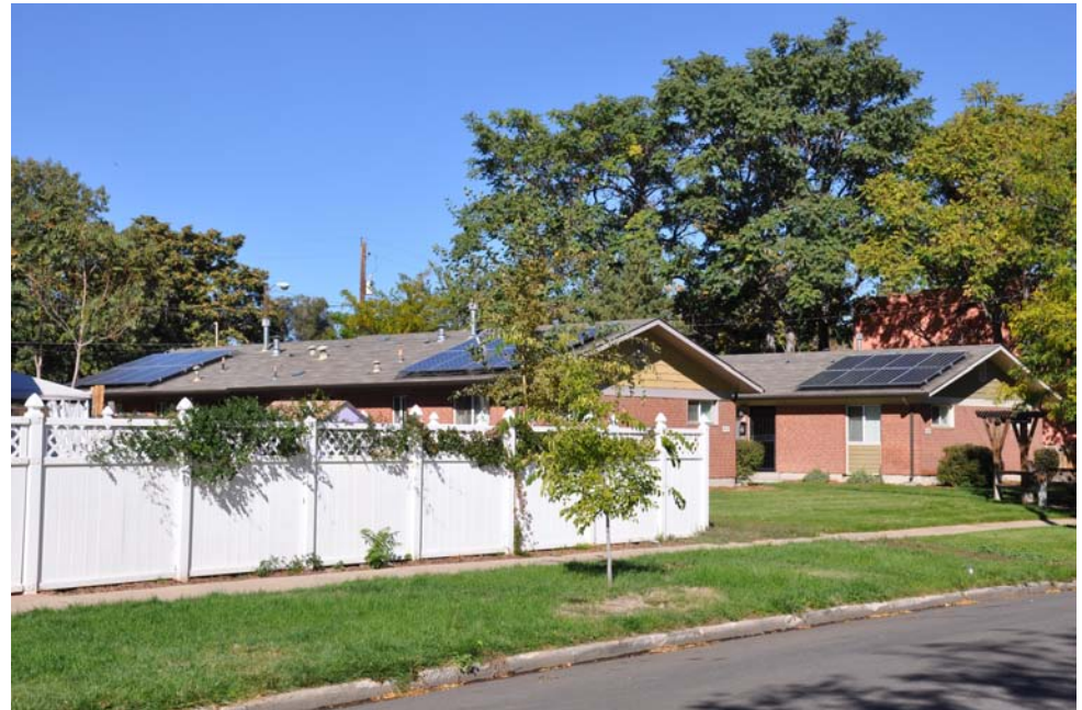
Northeast Denver Housing Center's Whittier Affordable Housing Project Source: NREL/DOE Image 19188
