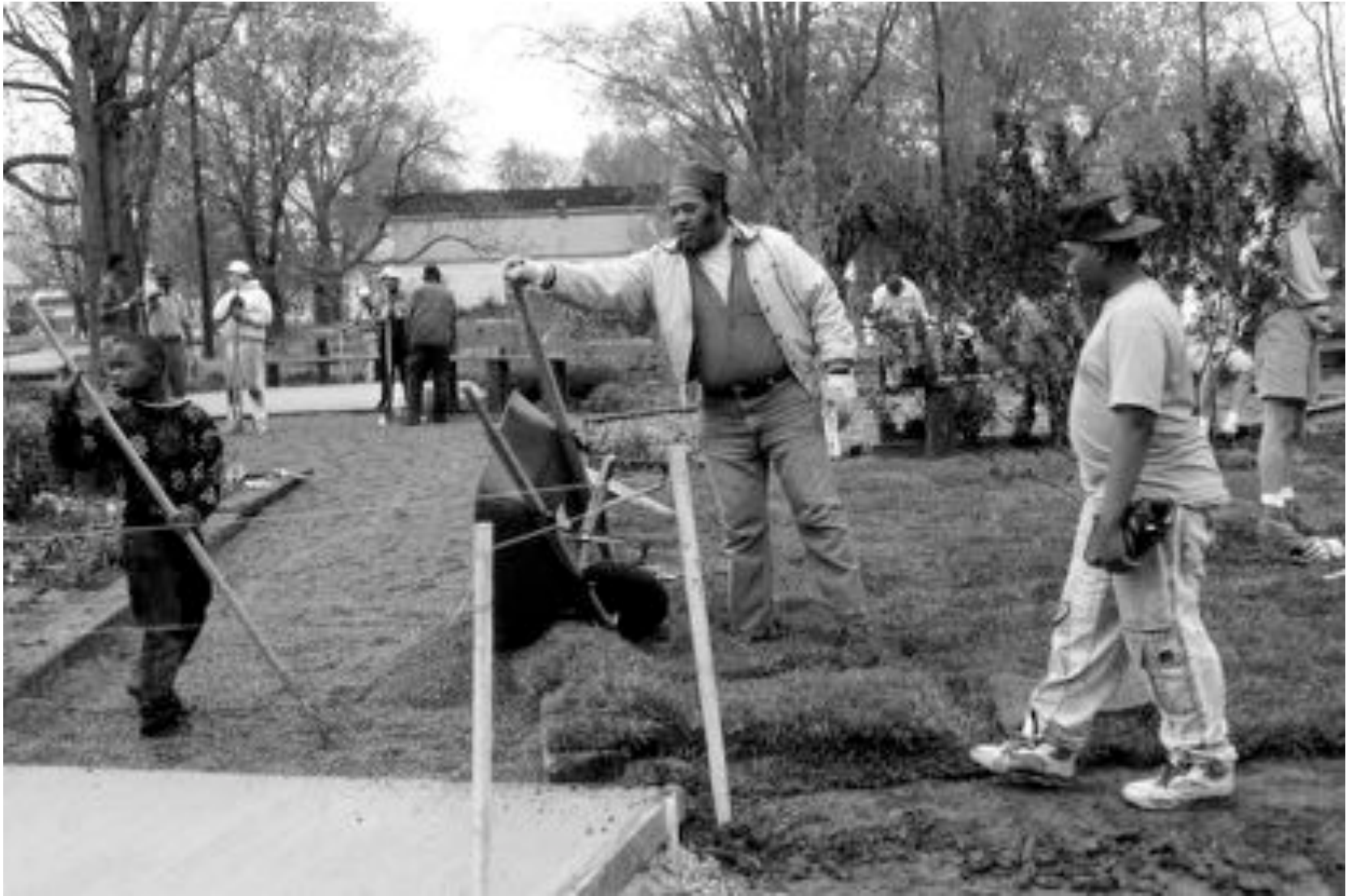
Construction of Illinois Avenue Playground
