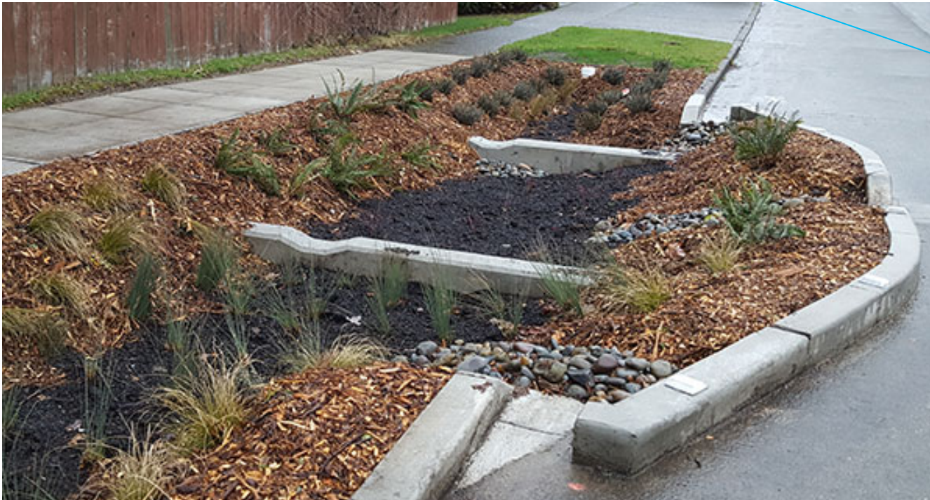
Natural drainage system cells and plantings in Seattle. Photo credit: Seattle Public Utilities.
